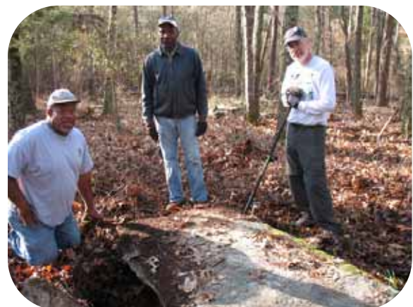
Volunteers reposition the top of a box tomb that had become dislodged due to a fallen tree
